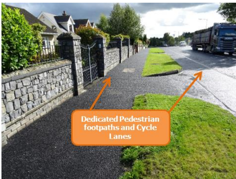
Figure 12.3 R407 Pedestrian and Cycle Facilities (Source: DBFL Site Visit Photograph)
